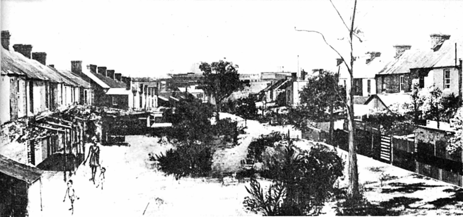
Artist's impression of what the community courtyard will look like when the project is completed. (Photo courtesy John Fairfax & Sons)
