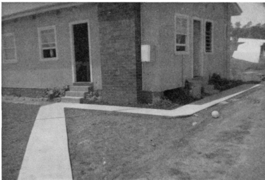
The new path laid to Mr. B. Toby's house on the Armidale reserve
