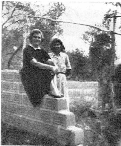
The unfinished wall provided an ideal perch for Victoria Lang, of Burnt Bridge, when she posed for her photograph with Yvonne Cochrane.
